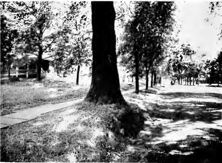
PLANTING SPACE INADEQUATE. SIDEWALK FORCED OUT OF ALIGNMENT AND GUTTER INVADED
